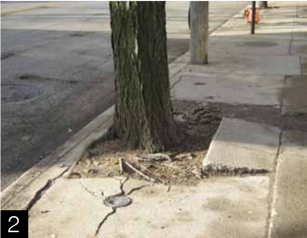
Photos: (1) A combination of obstacles on the sidewalk and little buffer between moving vehicles and sidewalks makes for an uncomfortable pedestrian zone. (2) Uneven walking surfaces and varied curb heights are hazardous to pedestrians.
